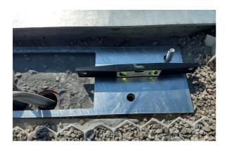
To tilt the floor plate, insert large washers below the floor plate until it becomes level.
