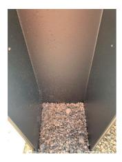
Depending on the subsoil, the size may vary. Please refer to the technical specifications of size and weight to determine and construct a solid foundation for the EV Base.
