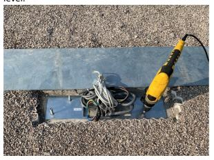
c. Mount the floor plate over the anchors and make sure it is level in both directions. If not, tilt the floor plate until it becomes level.
